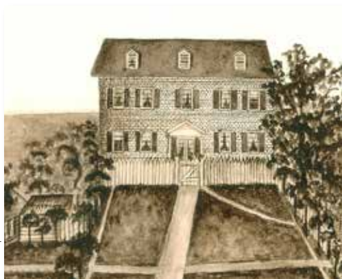
Original Building, Saint Michael, Louisiana, 1825
